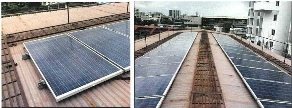
Plate 20 : Installed Solar PV panels on the sloping roof of the college
