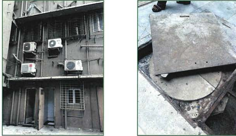
Figure 16: Rainwater harvesting down-take pipe and Recharge Ring well provision in campus
