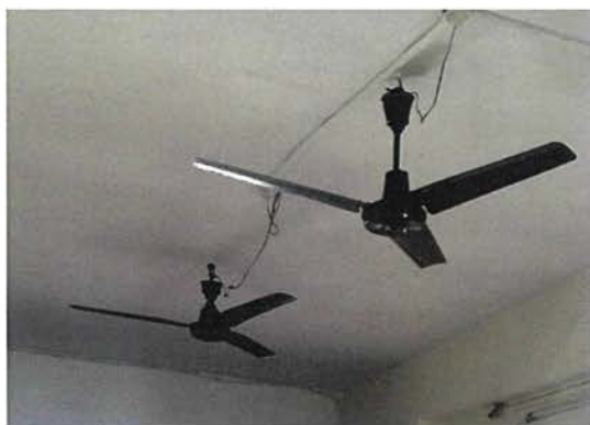
Plate 25: Existing Ceiling Fan of 60 W
