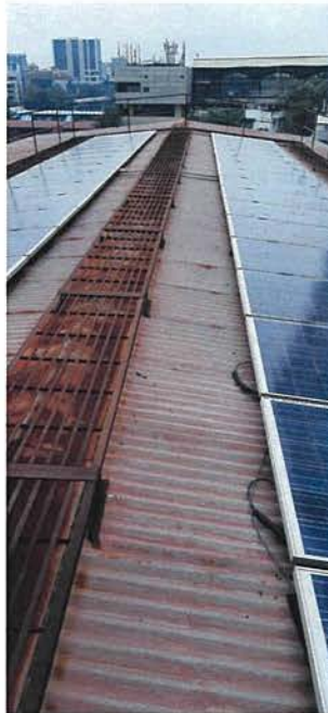
Figure 19: Picture showing the current gangway and open cables of the Solar PV panels
