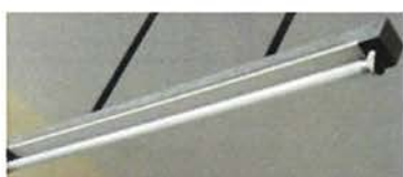
Plate 23: Existing 36W Fluorescent Tube Lights
