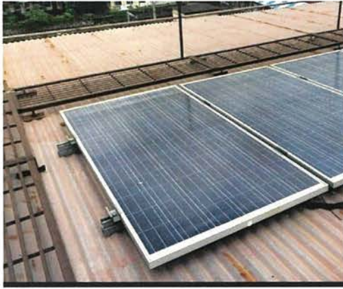
Plate 20 : Installed Solar PV panels on the sloping roof of the college
