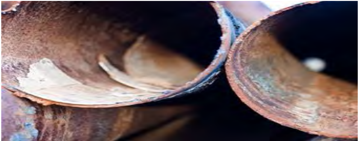
Fig.1.12: Oil and gas pipeline under sour corrosion [63].
