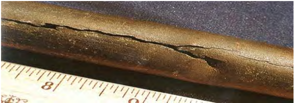
Fig.1.10: Oil and gas pipeline after being attacked by stress corrosion cracking [60].
