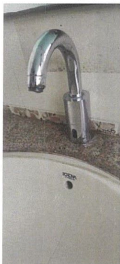
Plate 7: Faucet with sensor with aerator and dual flush
