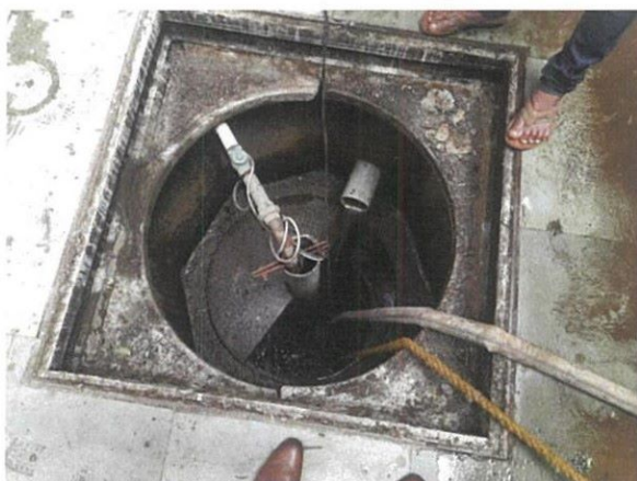
Plate 8: Rainwater tank with down take pipe
